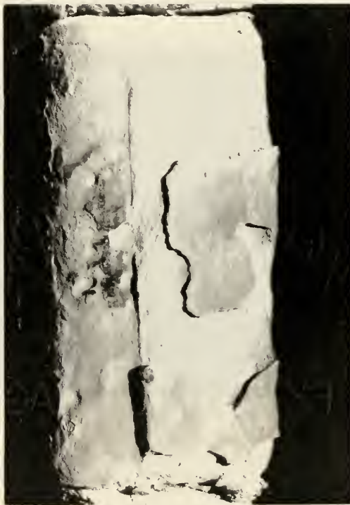
Fig. 24. Exfoliation of yellow sandstone at base of arch in east wall of nave (Photo: Anne Brackin)
